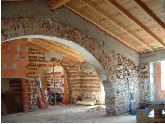
Madeiramento com painel sandwich
